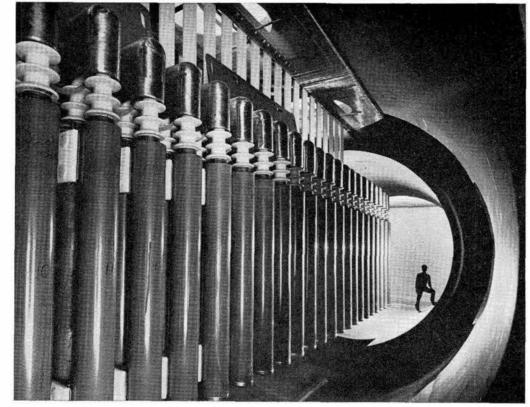
HERMES II capacitors will store a maximum of one million joules to provide the basic energy of the machine. Interior of steel tank will be filled with 150,000 gallons of mineral oil. Ray Clark is silhouetted at front of tube.
